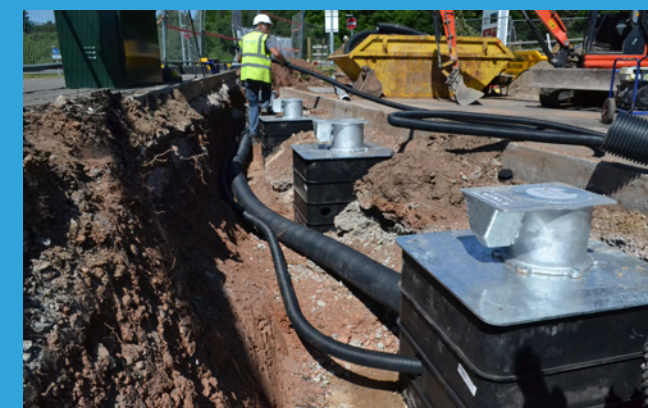
Civils infrastructure being installed
