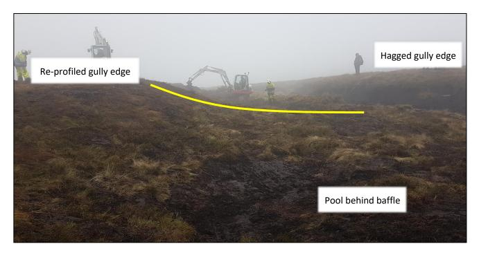
**Figure 3.7** | A peat baffle in a gully. An example of a peat baffle in the Brecon Beacons (the baffle is highlighted by the yellow line). This baffle is approximately four metres long and stretches across more than half the width of the gully. A small pool (less than ten centimetres deep) has been created behind the baffle to facilitate colonisation of peat-forming vegetation such as *Sphagnum* moss.
