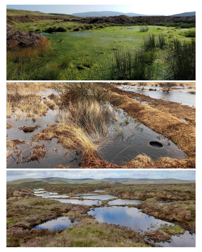
**Figure 3.5** | Wide gully dams Top: a wide 'leaky' peat dam at Blaen y Coed (Photo: Rachel Harvey, SNPA). Middle: a plastic pipe drainage hole installed into a dam – this right-angled pipe allows water to flow through the pipe to the bottom of the dam on the other side (Photo: Chris Holgate Contractors). Bottom: A gully blocked using a 'honeycomb' effect. This site is being restored with biodiversity and the bird assemblage in mind, so pools like this will be of great benefit.
