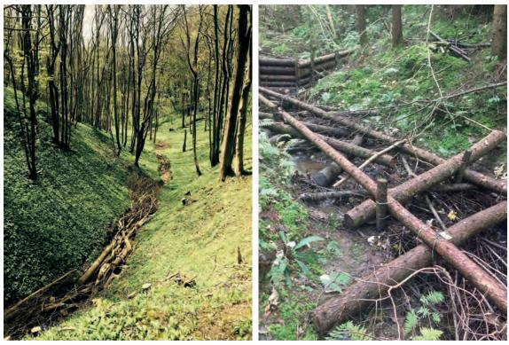
Figure 10.11 Gully stuffing (courtesy Marc Huband, Atkins) Figure 10.12
