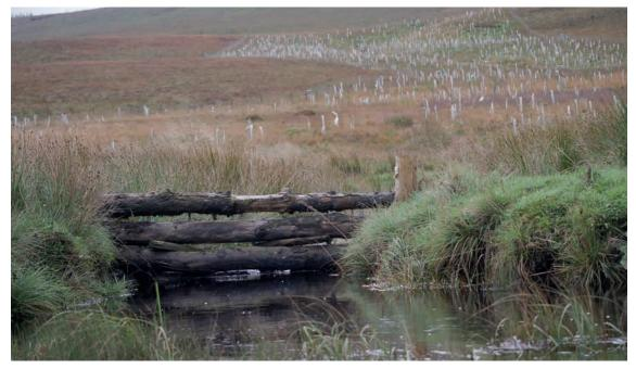
Figure 10.10 Stake and wedge leaky barrier (courtesy Yorkshire Dales Rivers Trust)
