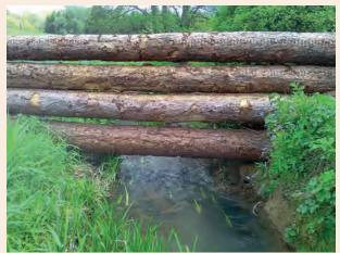
Figure A1.18 Updated leaky barrier designs from 2020 (courtesy Water Friendly Farming)
