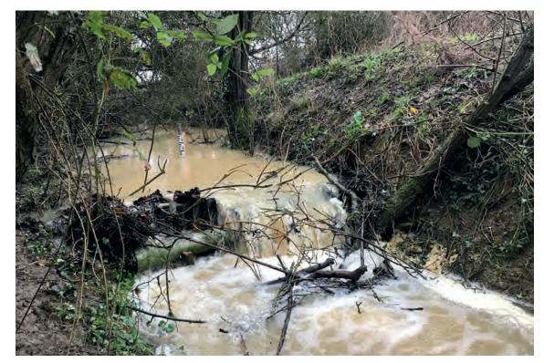
Figure 10.9 Banktop diverter or flow spreader/large log leaky barriers (courtesy Marc Huband, Atkins)
