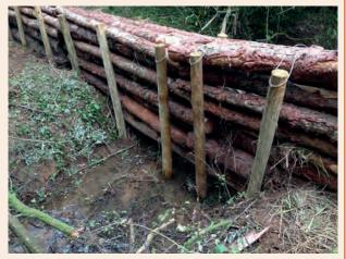
Figure A1.17 Initial leaky barrier designs from 2016 (courtesy Water Friendly Farming)
