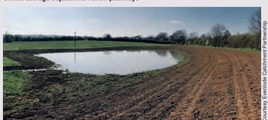
**Description:** areas that have been adapted to store water by diverting it from a runoff pathway, temporarily store it, and then slowly release water or allow it to infiltrate or evaporate after flood levels have receded.
