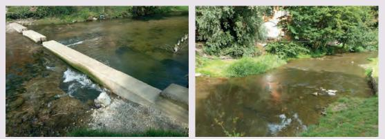
Removal of a failed weir structure (before and after) on the River Great Ouse, Buckingham (courtesy River Restoration Centre)
