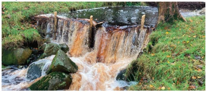
**Figure 3:** A leaky barrier in high flow conditions. A number of fascines (bundles) have been placed in the river to help slow the flow and store water behind the barrier during periods of heavy rainfall, helping to reduce downstream river levels. (©Sam Hope, Wyre Rivers Trust)
