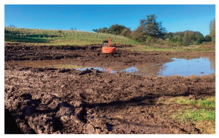
**Figure 15:** An excavator creating a large pond at the base of a slope, on which a woodland has been created. (©Sam Hope, Wyre Rivers Trust)
