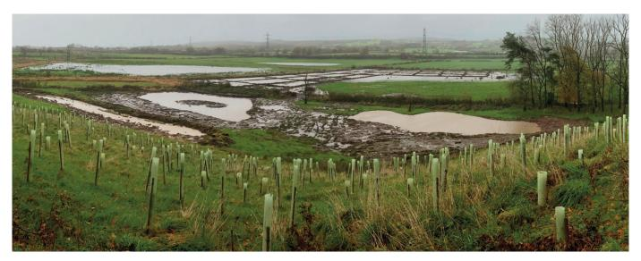
**Figure 4:** A panoramic view of a Wyre Natural Flood Management Project site. In the foreground is an area of woodland creation. Beyond that are two ponds created to store water from surface flows. In the background is an area of lowland peat restoration. All these interventions are helping to store water and restore critically important habitats. (©Sam Hope, Wyre Rivers Trust).
